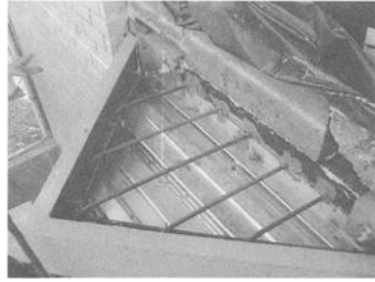
Figure 11 – Cantilevered slab extension at new endwall windows.
