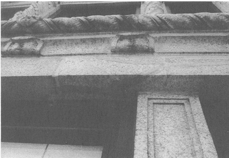
Figure 9 - Inappropriate Repairs
