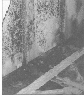
Figure 5 - Spall on interior side of stone panel at panel connection and corrosion of backup observed during survey of the interior side of the stone panels.
