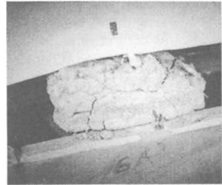
Expansive mortar used to set stone.
