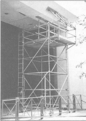
A. Installation of Shoring and Barricades
