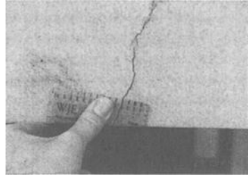
Crack measurement using a width gauge.
