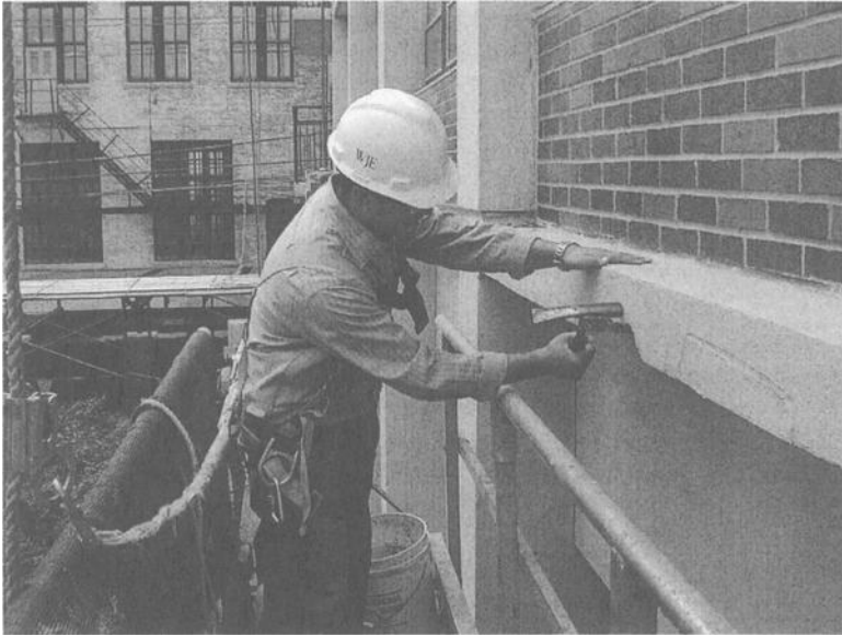
FIG. 7 - Sound testing of concrete with a hammer to detect delaminations.
