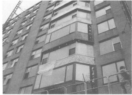
Figure 9 – Reconstruction Proceeded Bottom to Top
