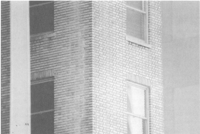
Figure 3 - Sealed Brick Cracks at the Building Corners
