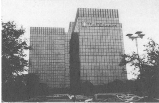
Photo 2 – Mottled appearance results from coating color changes
