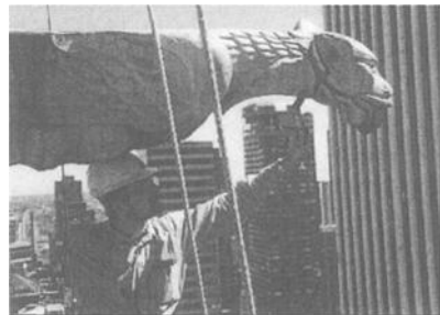
Sounding for internal defects.
