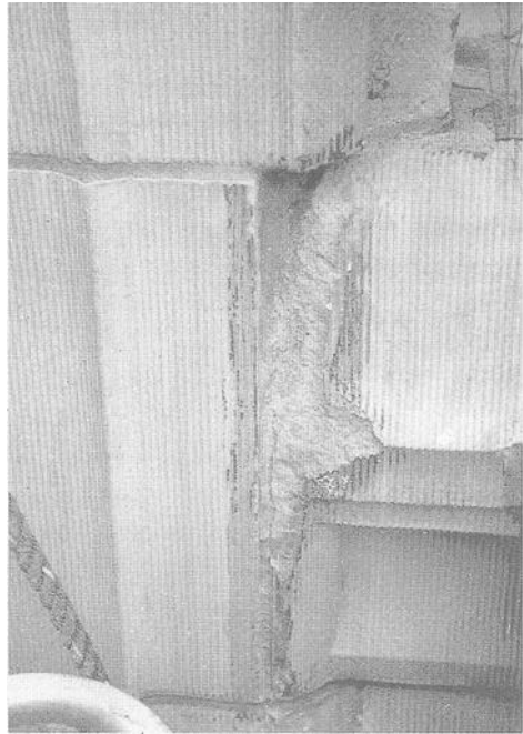
Figure 7 - Material Spall
