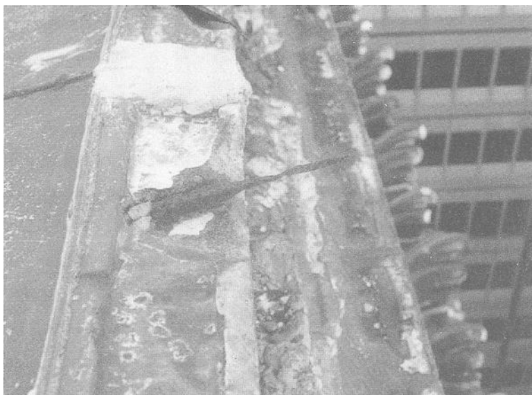
Figure 8 - Corrosion Failure
