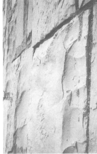
Figure 4 - Good continuation of the lines in this sedimentary stone camouflage separations in the stone’s layers.
