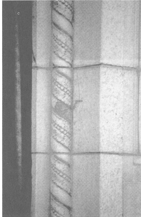
Figure 5 - Glaze Spall
