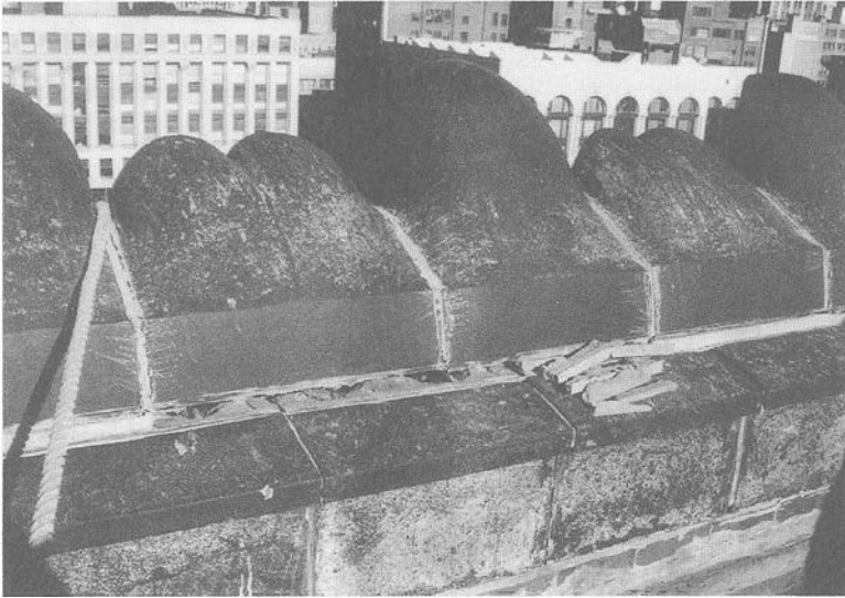
Figure 6 - Mortar Deterioration
