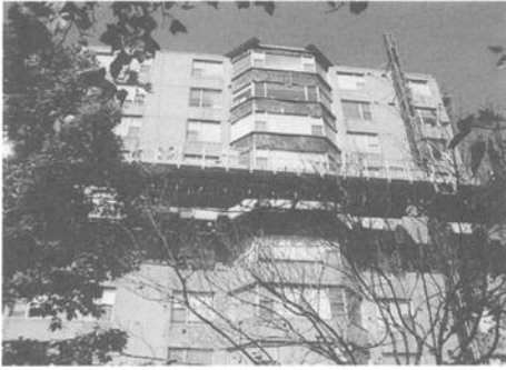
Figure 8 – Bay Demolition Proceeded Top to Bottom
