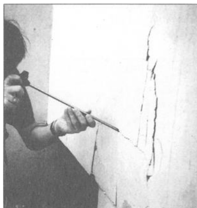
Figure 7 - Use of a borescope at a distressed limestone facade panel
