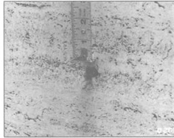
Figure 15 - Ferrous through-stone repair anchor
