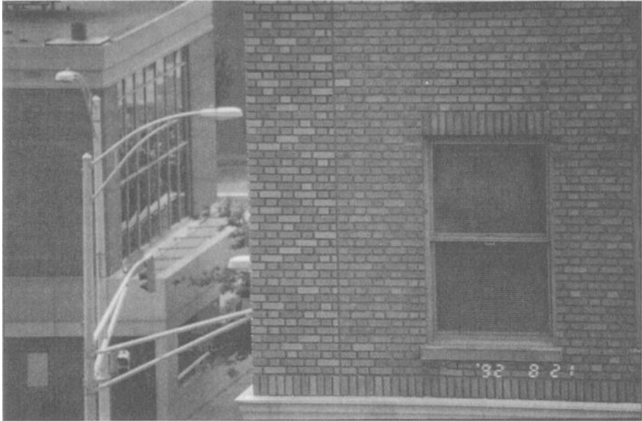
Figure 10 - Completed Corner Repair
